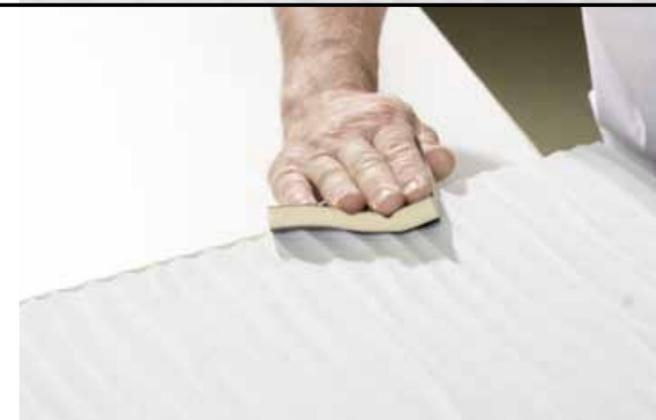
Finally clean structure oriented with a sanding pad (ap. grain 100).
