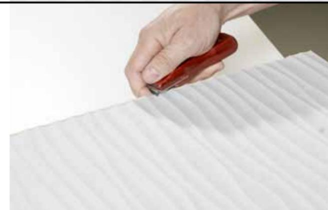
Finish the edge with a draw blade in a 90° angle to orientation of structure.
