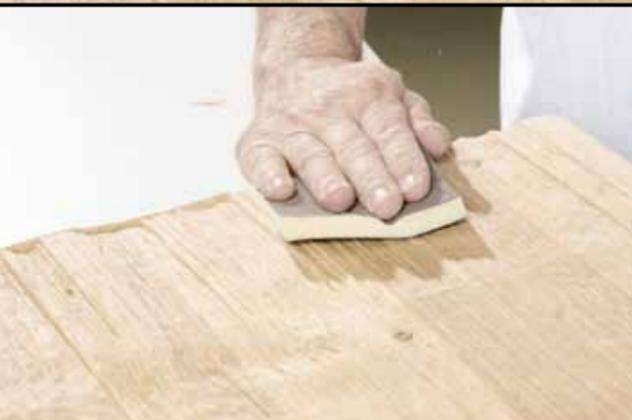
Grind the edge subsequently parallel to structure path with a sanding pad (ap. grain 100).
